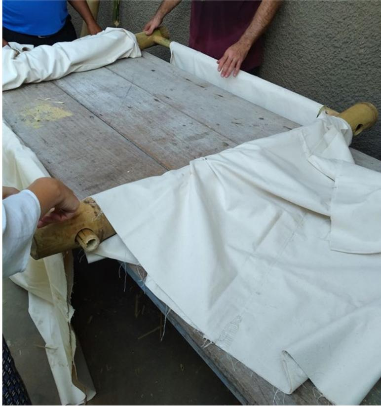
9. Load 4kg of stones into each thick base bamboo on both sides of the cane, making a total of 8kg of weight added for the structure
